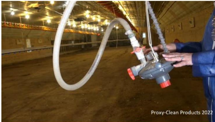
Step 5. Shut the regulator's valves off when the cleaning product filled into the system. Leave the product in the water
